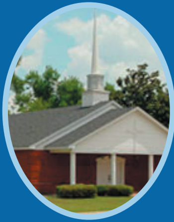
Foreman First United Methodist Church
